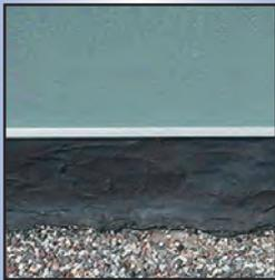
After - Installation of new Reinforced Perimeter Flashing Strip with butyl tape attached and EPDM flashing. New EPDM flashings are seamed to the underside of the existing EPDM field membrane.
