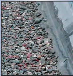
Before - Tenting of EPDM membrane at perimeter wall due to loss of attachment of membrane to base tie-in.
