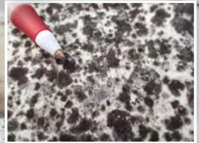
**Photo 1** Biological growth has impeded full drainage. Reflectivity typically suffers in these areas
